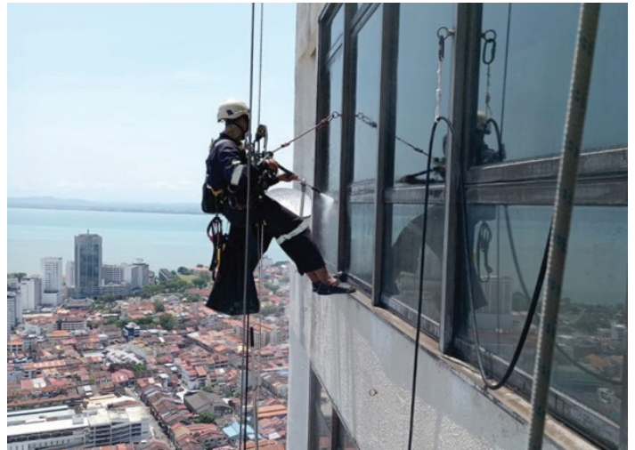
Kerja pembaikan rekahan dinding | Wall crack repair work
