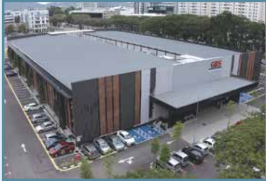
GBS @ Mahsuri building drone
