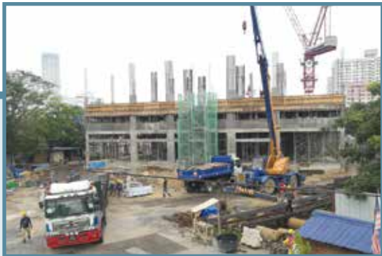
Structural Works In Progress For Level 2 - Cecil Residency, Georgetown
