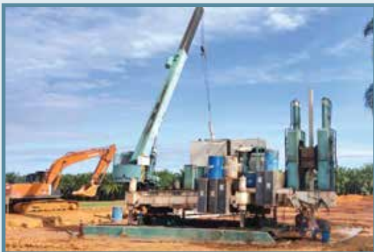
Earthworks In Progress - Ladang Byram, Nibong Tebal
