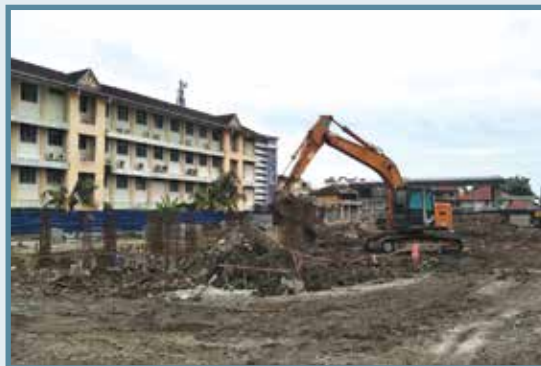
Structural Works In Progress For Level 1 - Mak Mandin, Butterworth
