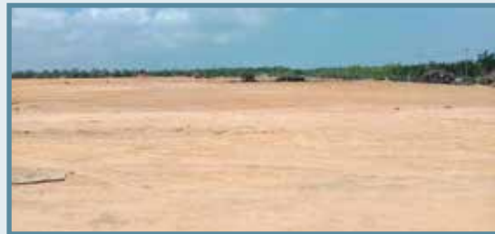
BKIP 2 Phase 1 Industrial Site
