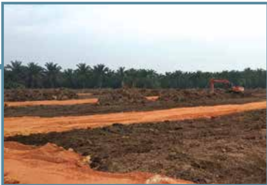
Striping Topsoil Work - Jalan Sungai Daun, Nibong Tebal
