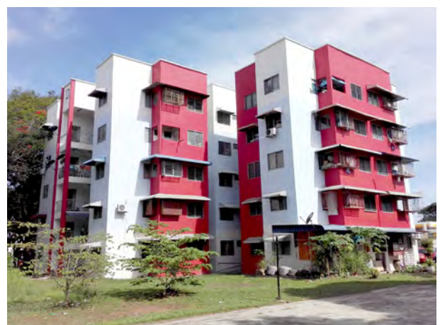
> Repainting Works at Bandar Seberang Jaya
