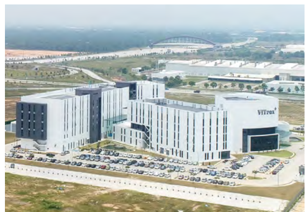
> ViTrox at Batu Kawan Industrial Park
