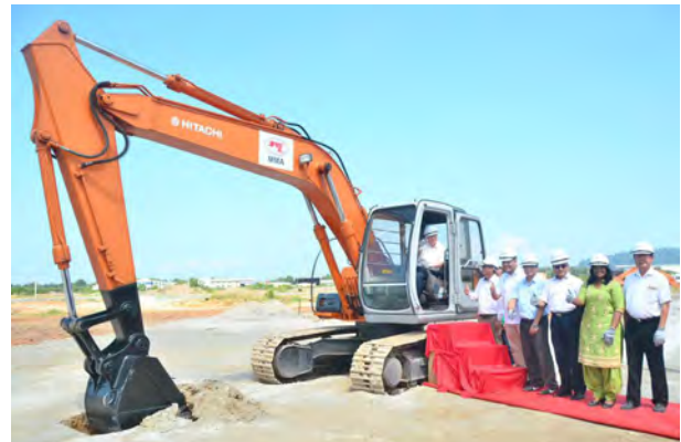
> The launching of road connecting Penang Science Park and Juru
