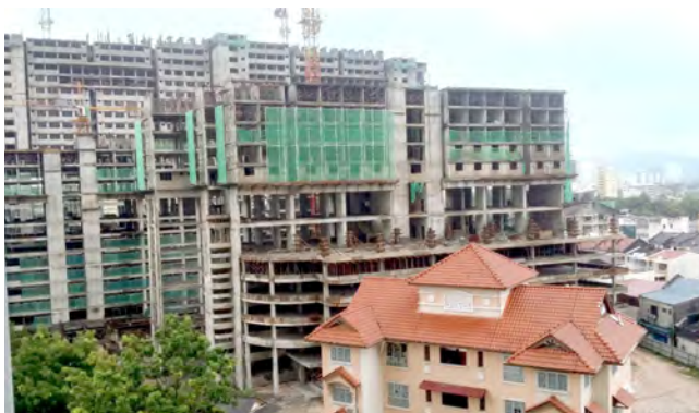
➤ Affordable Housing Project at S P Chelliah by Zubicon Sdn Bhd
