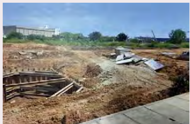
Site works at North Penang Science Park
