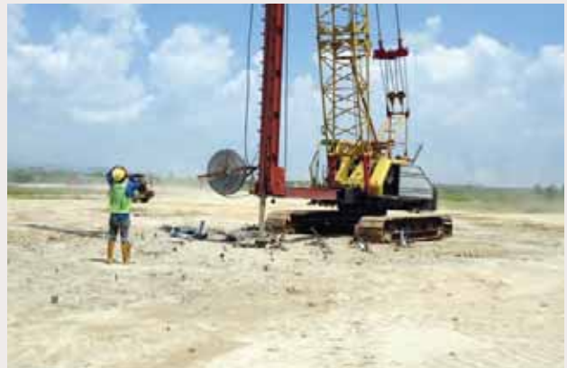
Perforated vertical drain works in Batu Kawan
