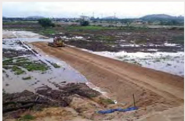
Infrastructure works at AHS, Phase 1
