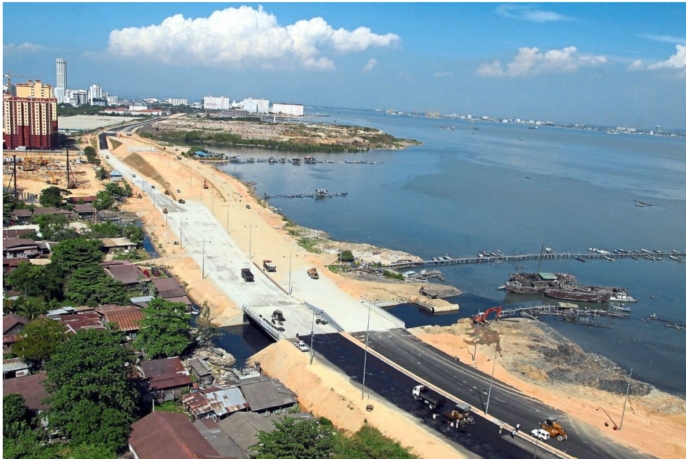
The Tun Dr Lim Chong Eu Expressway in Jelutong under construction in January 2003. To date, almost the entire east coast of Penang island has undergone reclamation.
