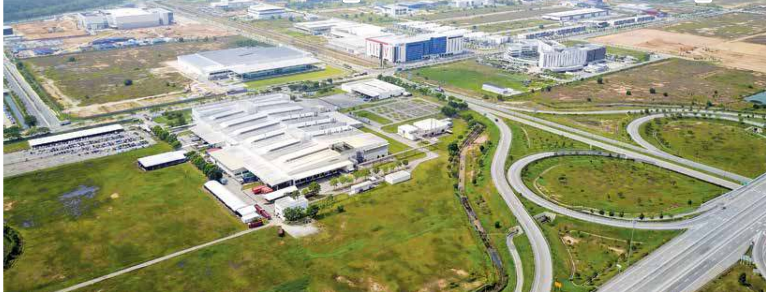
The view of Batu Kawan Industrial Park from the sky and the infrastructure network that PDC has built to enhance the connectivity of Bandar Cassia.
